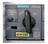
Transformer circuit breaker for Measurement & Control Unit (MCU) (=EIN-1Q2) (illustration similar)
