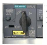
Transformer circuit breaker for Measurement & Control Unit (MCU) (=EIN-1Q2) (illustration similar)
