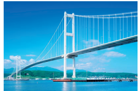
• 桥梁与大坝监测 Bridge and dam monitoring
