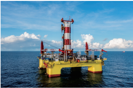
• 石油钻井设备位移反馈 Oil Drilling Equipment Displacement Feedback
