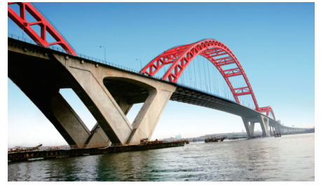
• 桥梁监测 Bridge monitoring
