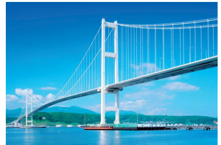
• 桥梁与大坝监测 Bridge and dam monitoring
