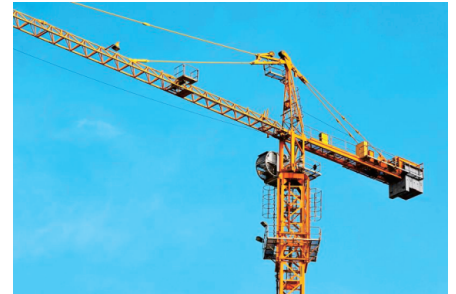
• 塔杆倾斜监测 Tower tilt monitoring
