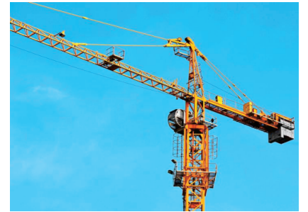
• 塔杆倾斜监测 Tower tilt monitoring
