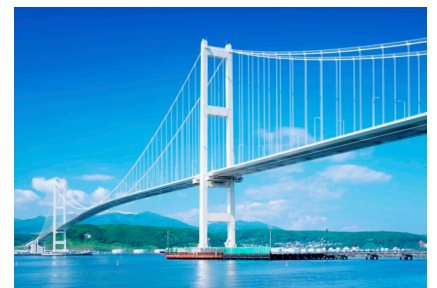
● 桥梁与大坝监测 Bridge And Dam Monitoring
